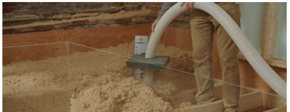
Direct placement method providing better control ►
