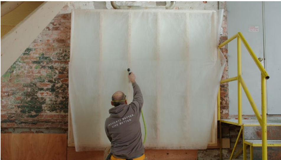
◀ Air permeable webbing being installed on the face of wall framing
