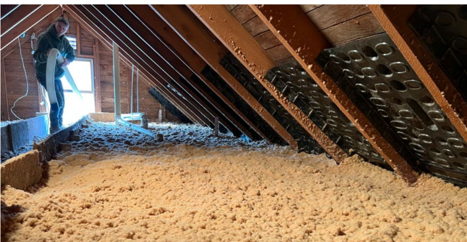
◀ Creating a dense attic blanket in a ventilated roof assembly
