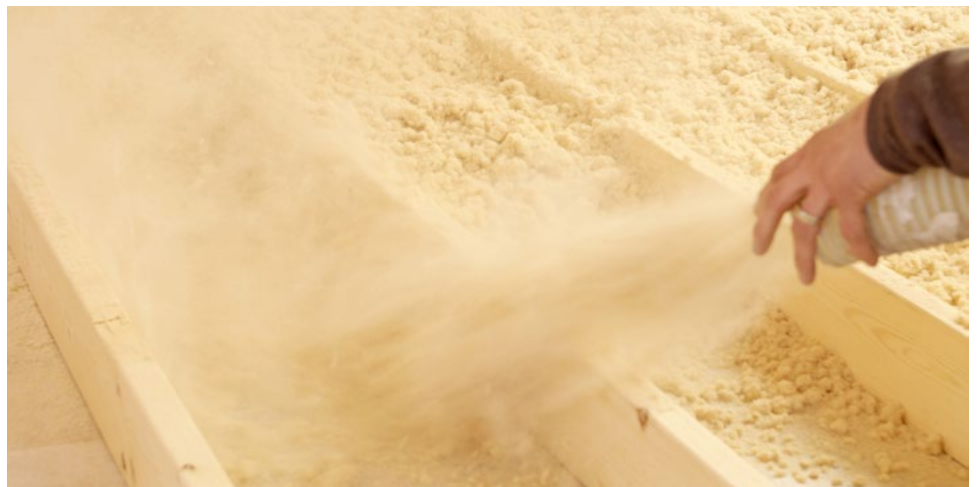
Installation in an open attic ►
